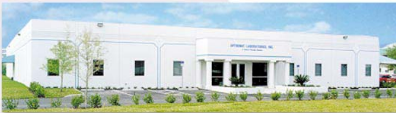
OPTRONIC LABORATORIES, INC. HEADQUARTERS • Orlando, Florida
